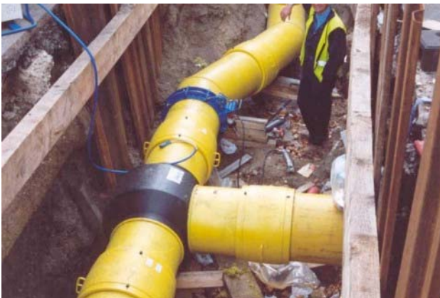
Picture 4: T-piece d 630 mm (British Gas)
